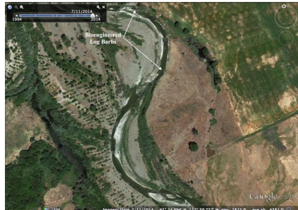
Image 7: River Mile 48 East Bank also showing boundaries of bank stabilization project, 2014 (Google Earth Imagery).
