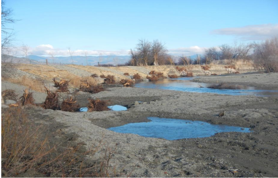
Photo 3: Completed bank stabilization at River Mile 36, November 2013 (Siskiyou RCD).
