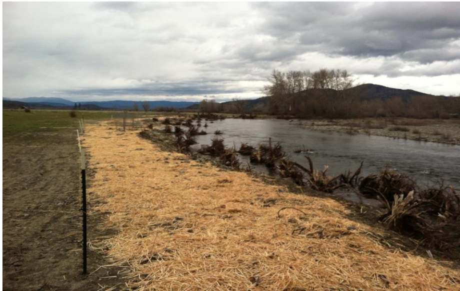
Photo 8: Completed bank stabilization at River Mile 52 looking downstream, December 2014 (Siskiyou RCD).
