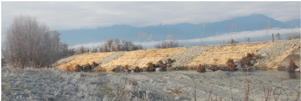
Photo 4: Completed bank stabilization at River Mile 36, November 2013 (Siskiyou RCD).
