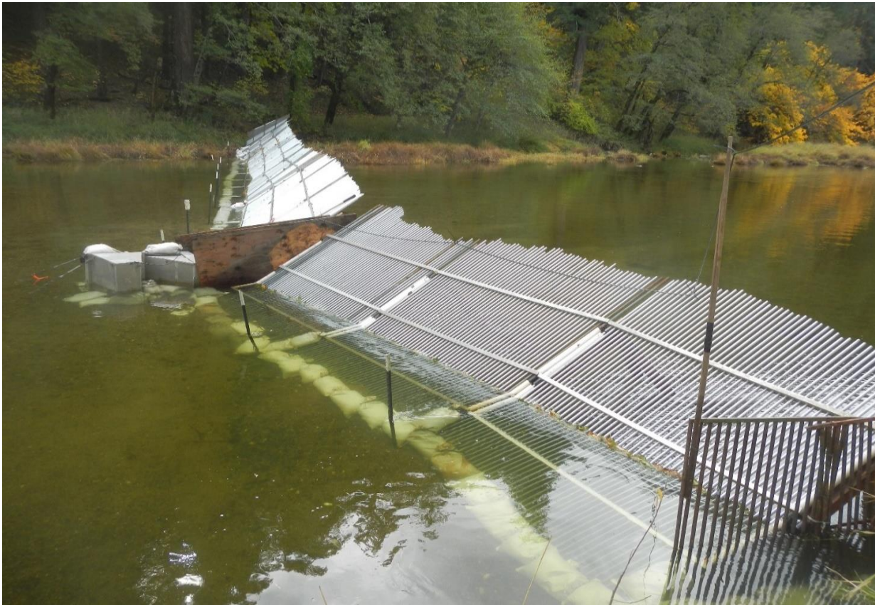
Figure 3. Scott River Fish Counting Facility located in Siskiyou County, California 2021.
