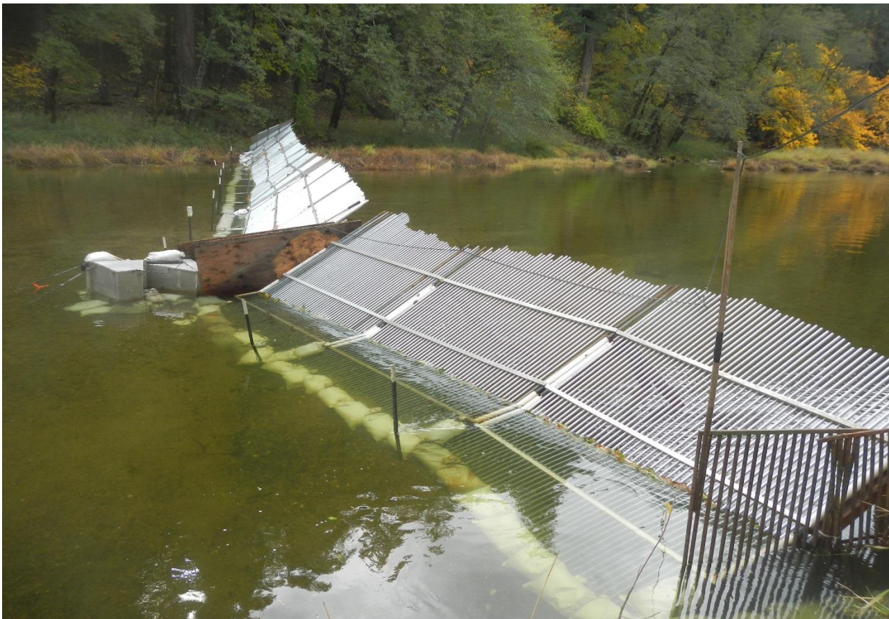
Figure 2. Scott River Fish Counting Facility located in Siskiyou County, California 2017.
