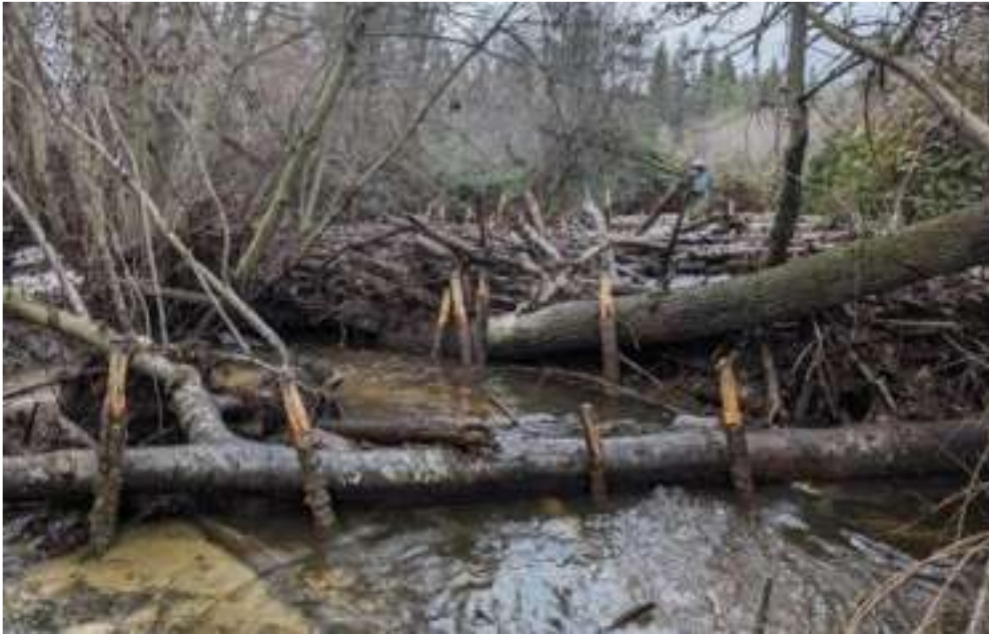
Photo 5. Log Jam looking upstream from mid channel with vertical logs placed to add support. December 21, 2023.
