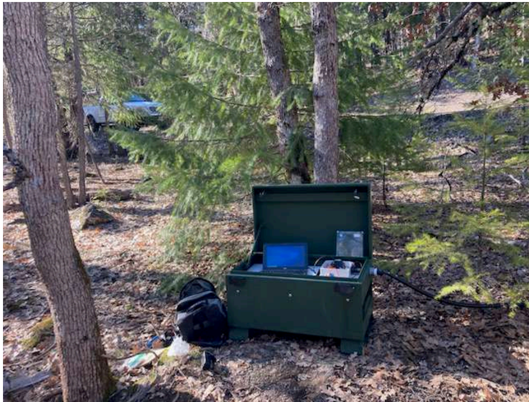
Picture 4. Data logger and power station at Scott River weir array.
