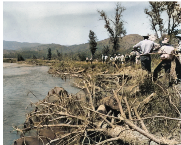
Tree rip-rap along Scott River. There were a total of six irrigation wells in the valley at this time. Photographer: Tumelson. May 12th, 1954.
