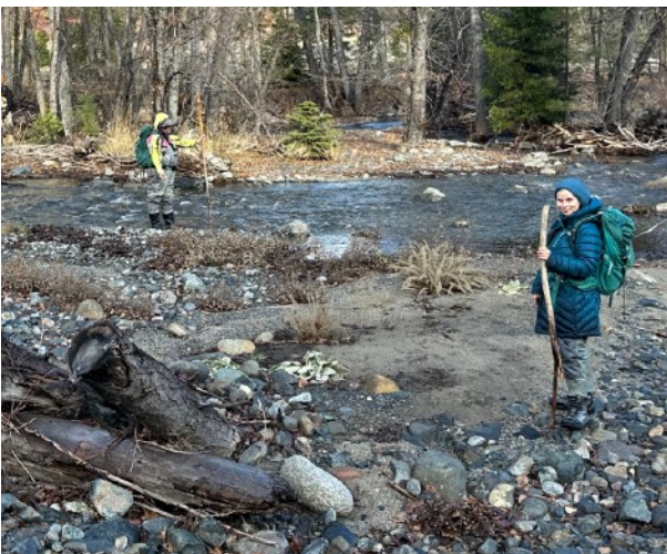
Tree rip rap along Scott River. Vegetation has been planted on bank to give added protection. 2023.
