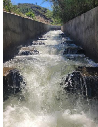
Photo 12. Flash boards (top) and view from downstream end of ladder (bottom) at 1.85 cfs (left), 4.47 cfs (middle) and 7+ cfs (right).
