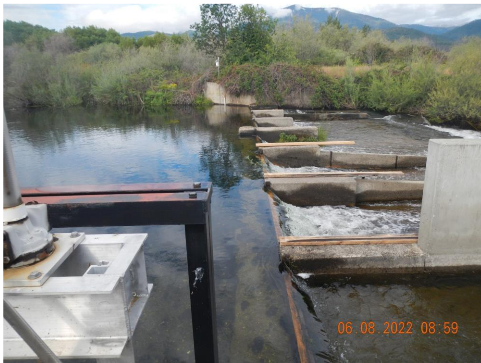
Photo 1. Young's dam with the headgate to the Scott Valley Irrigation District ditch in the left foreground, upstream end of fish ladder in the right foreground, and concrete apron with dam board slotst extending across the main channel.
