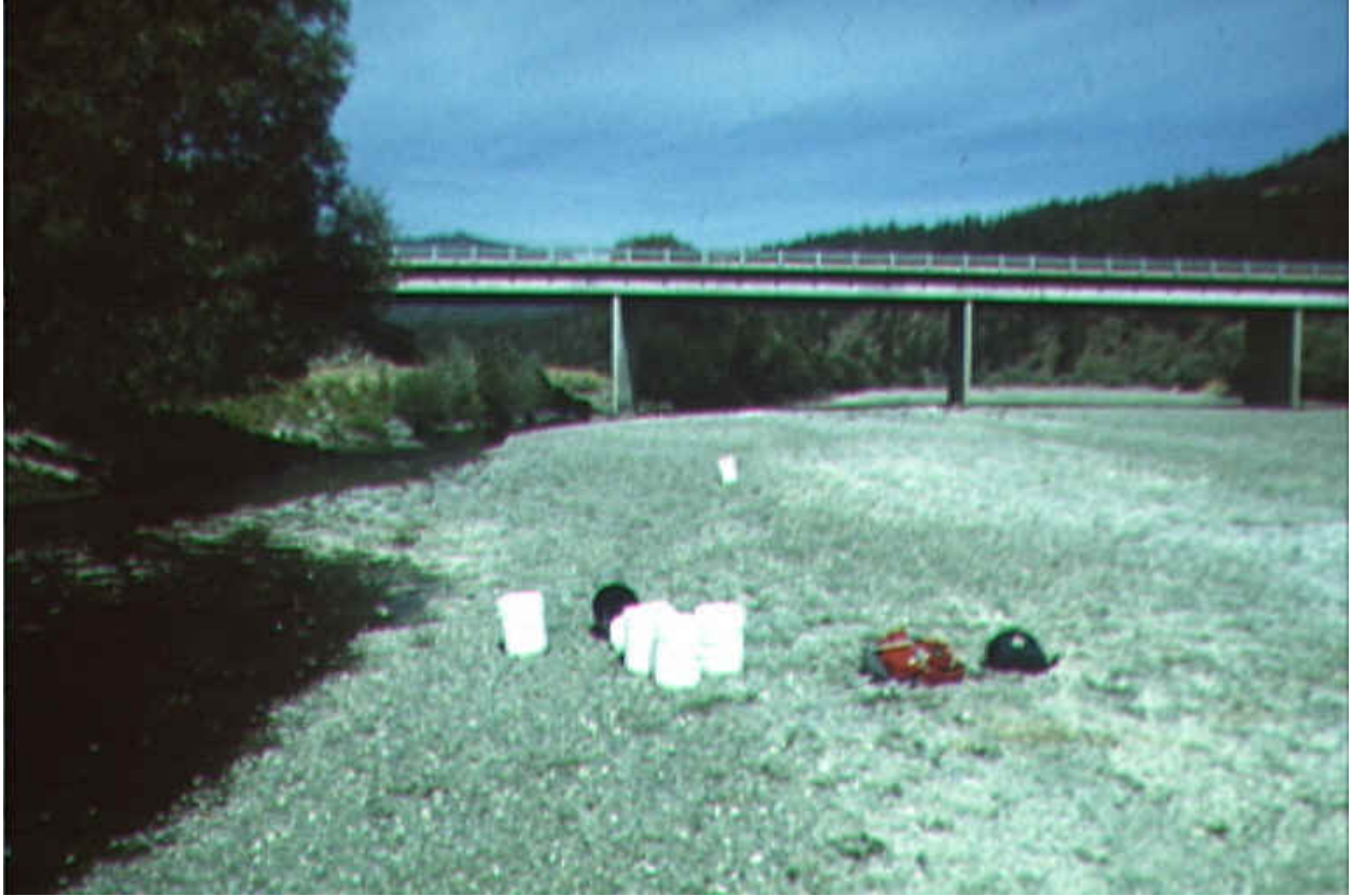
Figure 2-A. Site B - 1989 Sampling - Meamber Bridge – Tozier
