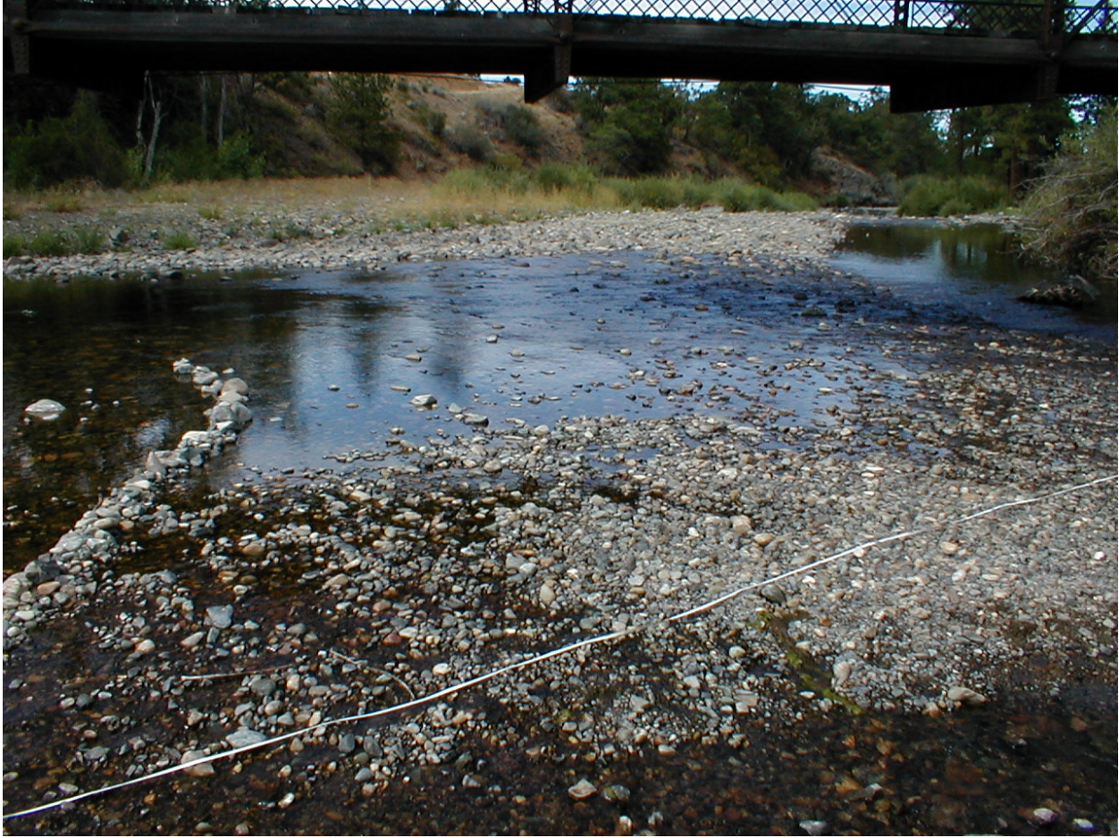
Figure 7-A. Site K- 2000 Sampling Site – Hayden. Near Red Bridge. Upstream view.
