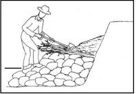
The above figure shows a brush layer being installed over a stone toe. Since the stone is not keyed into the bed, additional stone is placed in the toe. As the bed is scoured adjacent to the bank protection, this additional stone is available to launch into the scour hole.
