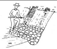
The above figure shows a verticle bundle being installed under a stone toe. The bundles are placed in trenches which are then filled with soil. This minimizes potential damage to the live material during stone placement as well as maximizes soil to stem contact.
