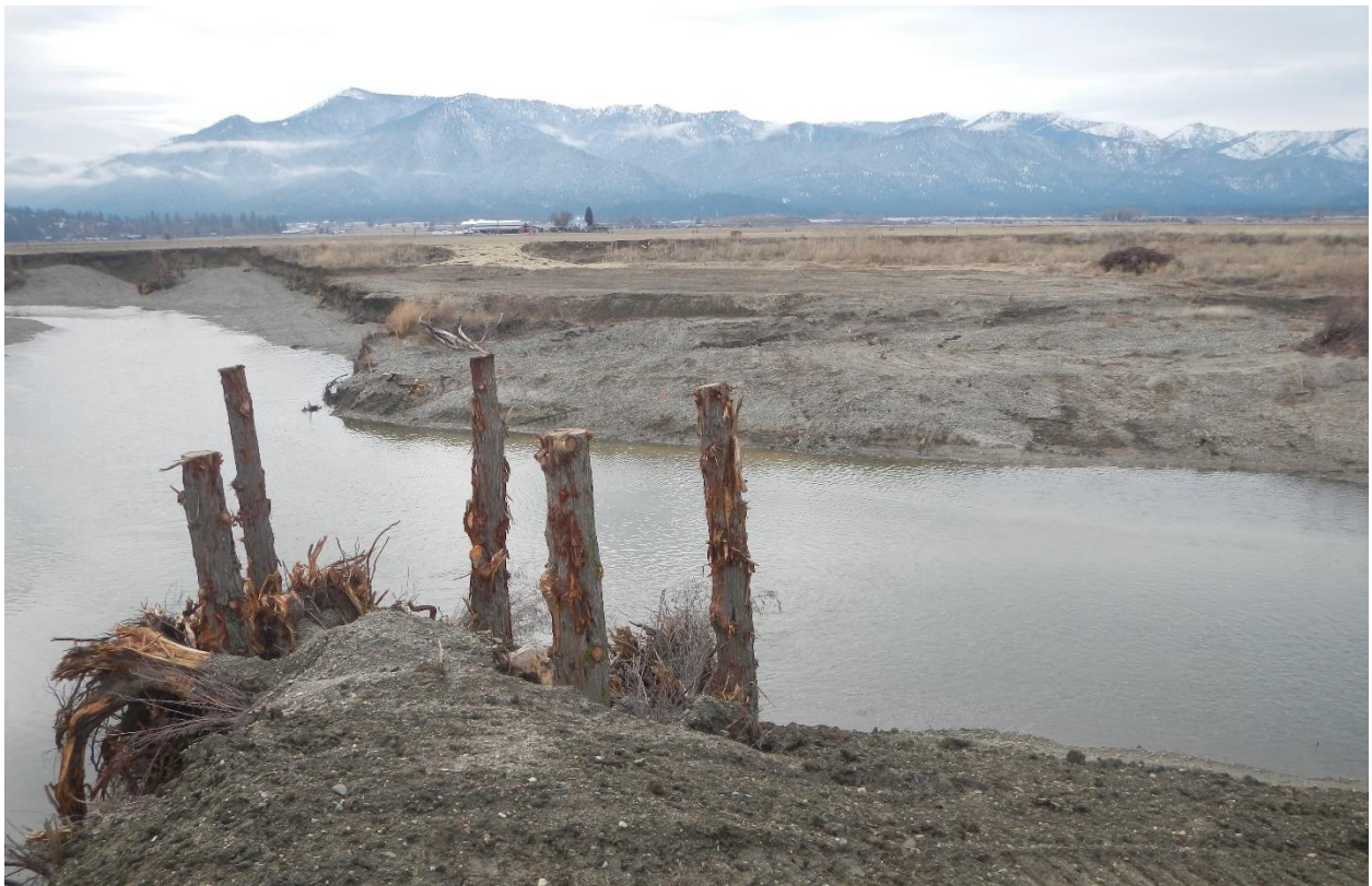
Figure 12. Western terraces and floodplain after re-grading, 12/4/18.
