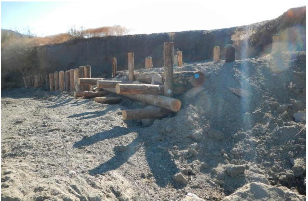
Figure 27. Type B ELJ after construction (western bank), 10/30/20.
