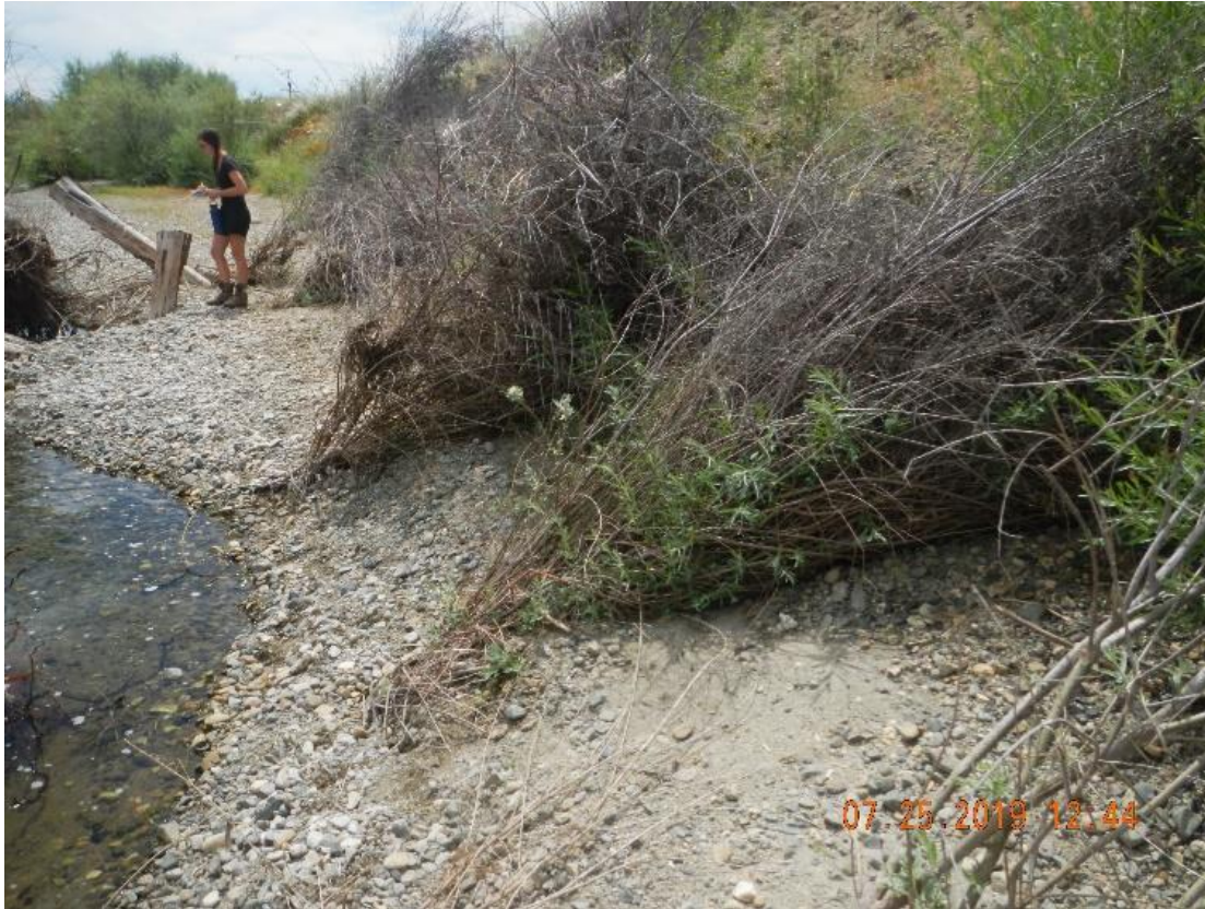
Figure 15. Willow clumps and bundles along the bank in association with the Type C ELJ, 7/25/19.
