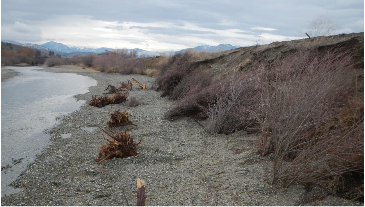
Figure 9. Type C ELJ after construction (western bank), 12/4/18.
