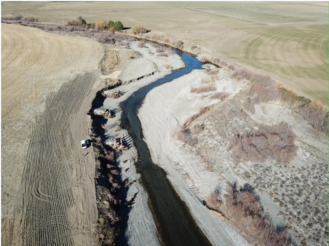
Figure 8. Scott River rkm 67 (looking downstream), 11/5/18.
