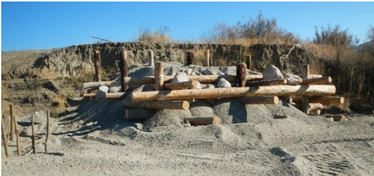
Figure 25. Type B ELJ after construction (eastern bank), 10/30/20.
