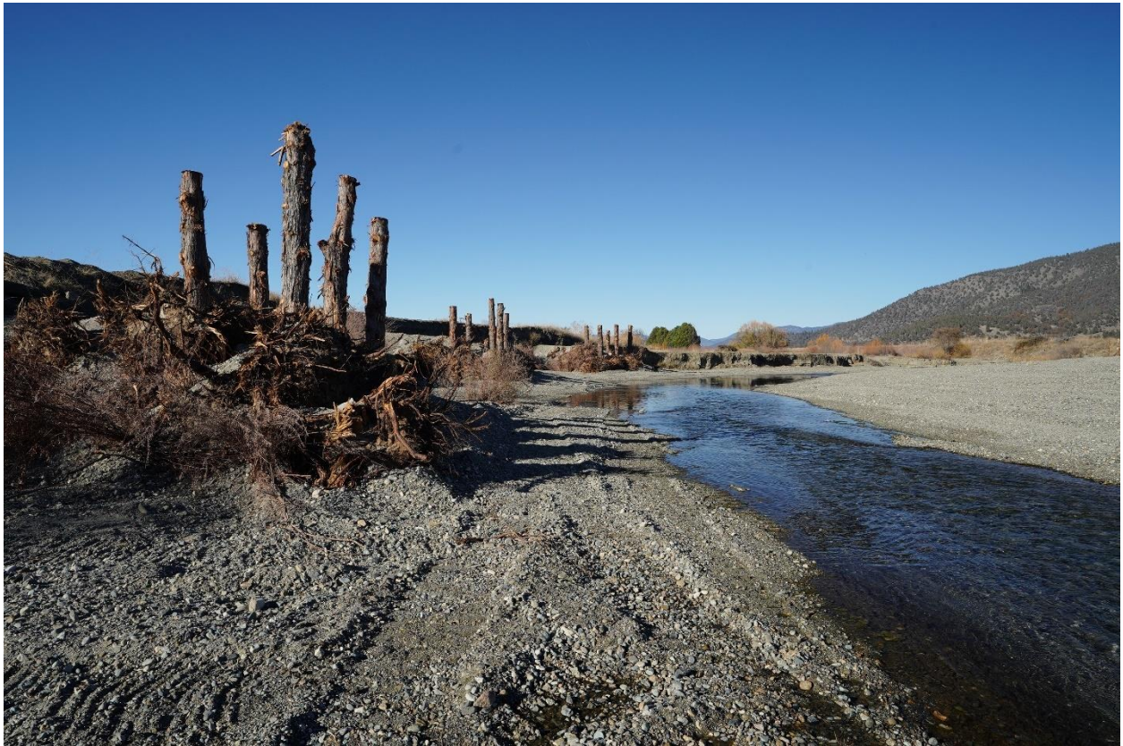
Figure 10. Type B ELJs after construction (western bank), 11/5/18.
